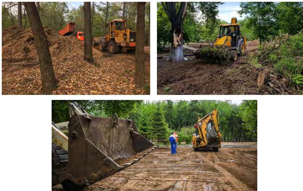
Figure 4.2.3.4.8. The use of heavy equipment in the upgrading of green areas. Work is carried out during the nesting period
