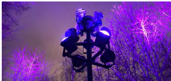
Figure 4.2.3.4.7. One of a thousand of pole-mounted floodlights installed in the PA "Vorobyovy Gory" ahead of the 2018 FIFA World Cup
