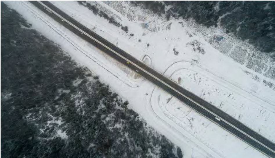
Figure 4.2.3.3.4. A section of the Central Ring Road in New Moscow 24
